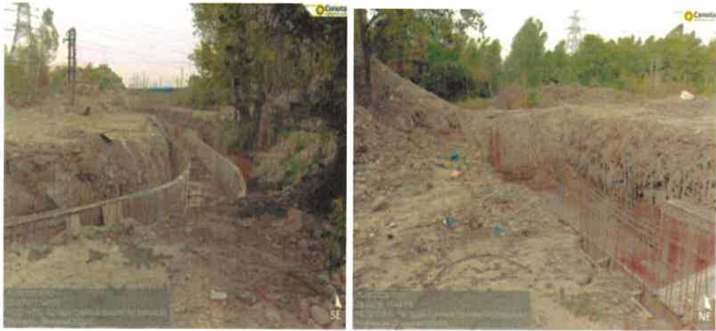
Figure:- Construction of drain.
