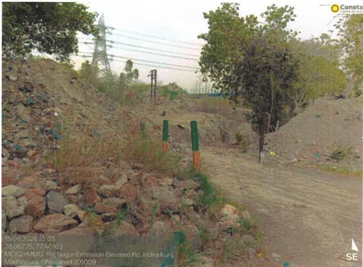
Figure:- Heap of Soil after digging drain
